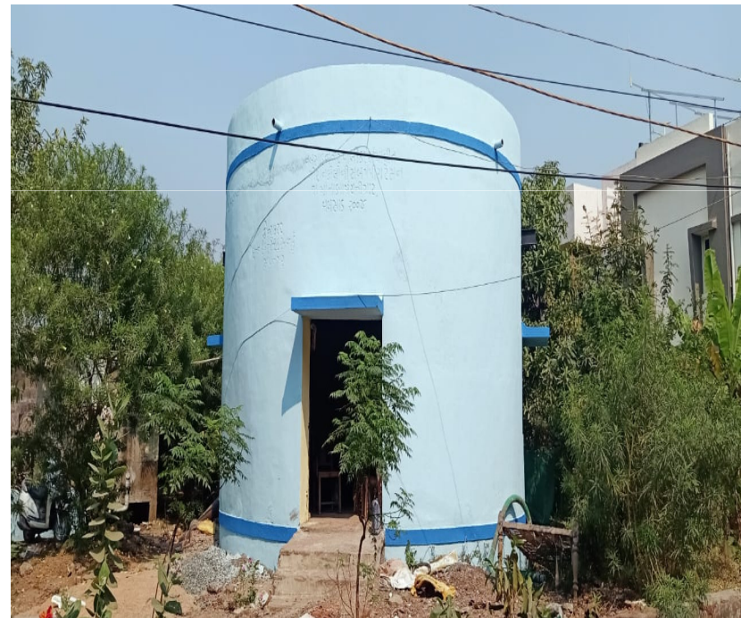
AmbuNagar Pumping station
